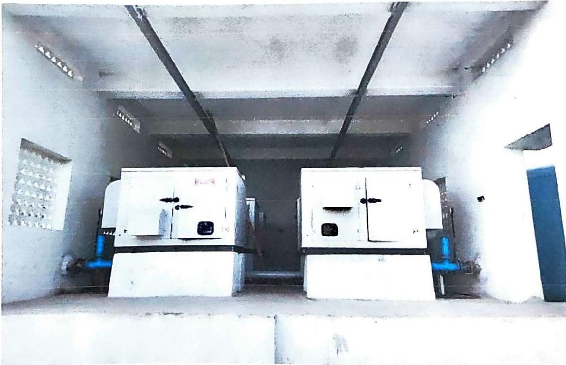
SUMP CUM PUMP HOUSE for Tertiary treatment Completed
